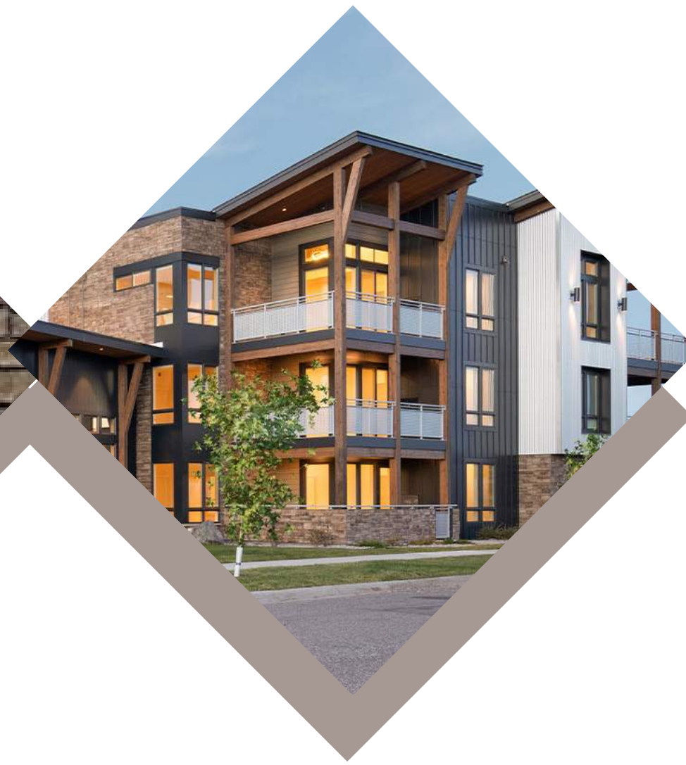
WOOD BEAMS & COLUMNS
