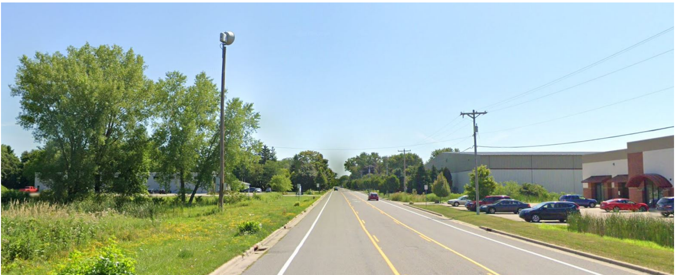
VIEW FROM VOGES RD LOOKING EAST
