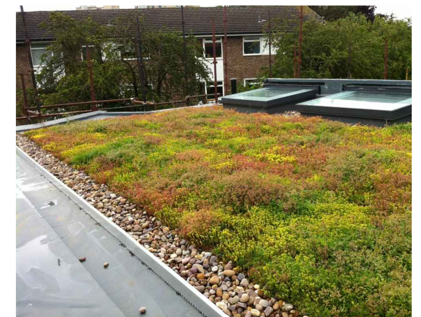
FULL SUN SEDUM CARPET GREEN ROOF WITH BALLAST EDGING - SEE PLANTING PLAN FOR MORE INFORMATION
