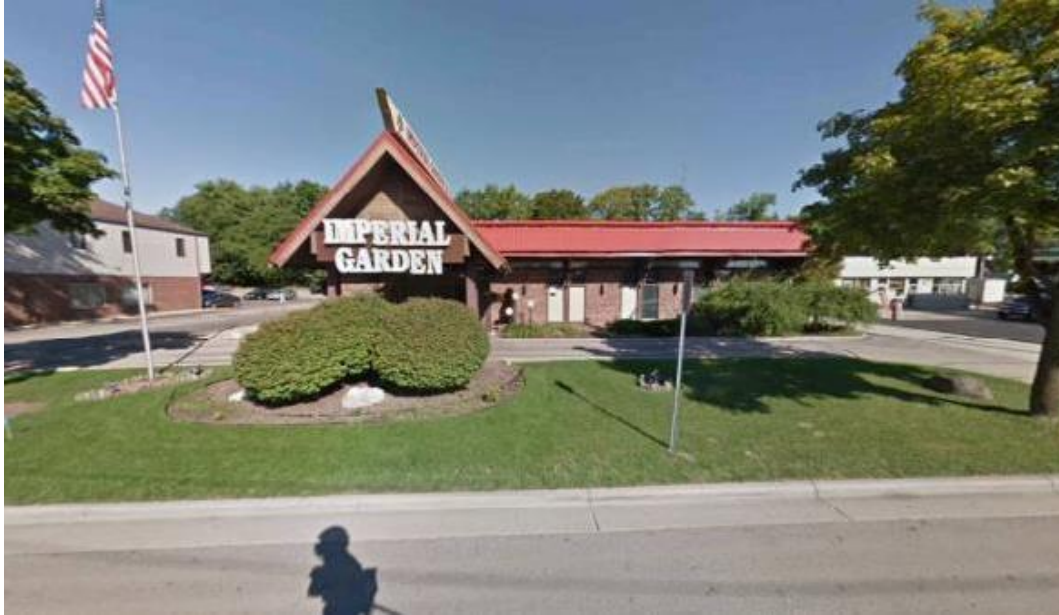
VIEW OF EXISTING BUILDING Viewing NW from Service Road
