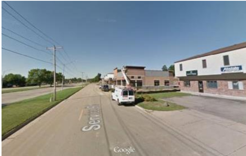
VIEW ALONG SERVICE ROAD Viewing SW, Washington Blvd. on left
