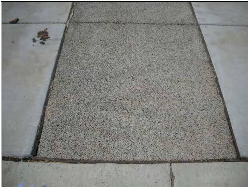
Photo 1: Close-up of permeable concrete compared to regular concrete.
