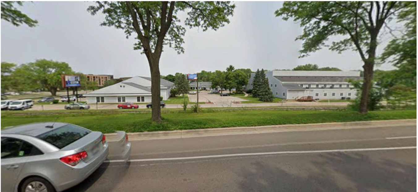
Old Middleton Rd (buildings to be demolished)
