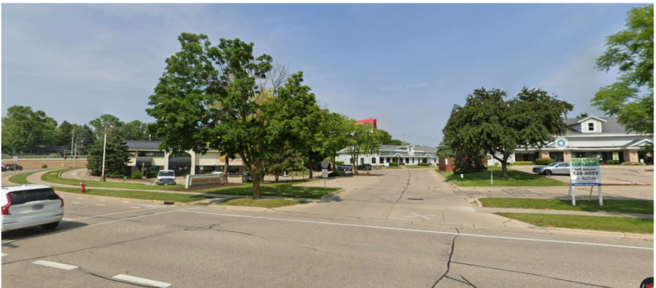
N Whitney Way (building to be demolished)
