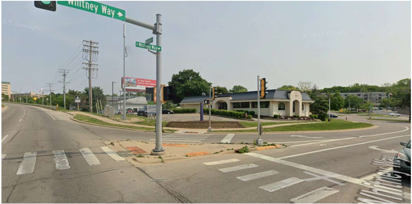
University Ave & N Whitney Way (building to be demolished)
