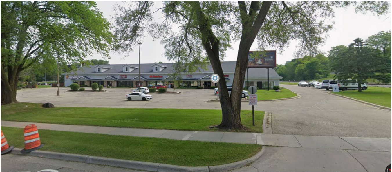
N Whitney Way (building to be demolished)
