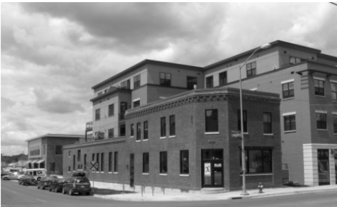
Figure D4: Variation in Roof Lines
