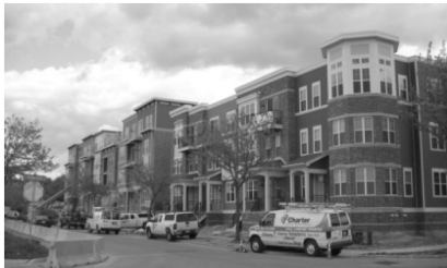
Figure D6: Building Alignment
