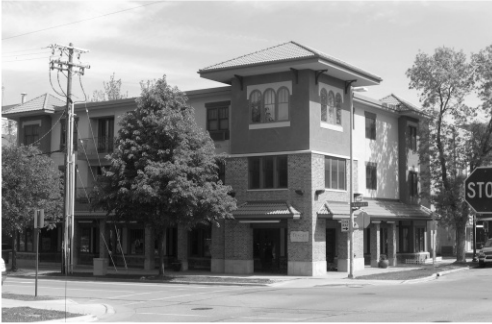
Figure D1: Entrance Orientation
