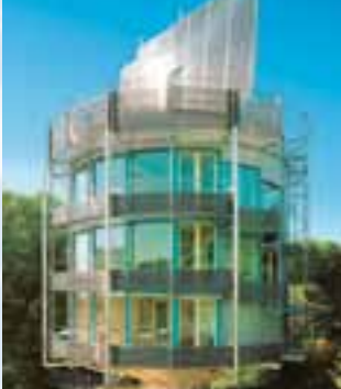
The Heliotrope – a rotating solar ‘tree-house’ which follows the movement of the sun
