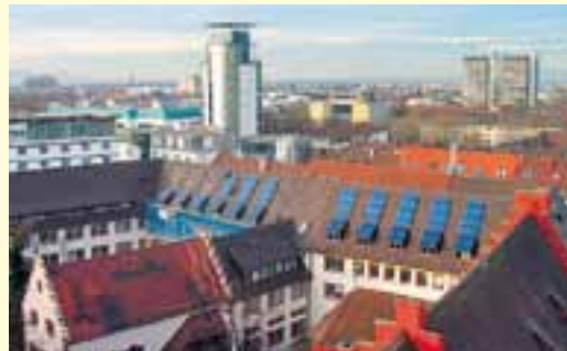
Solar City Hall
