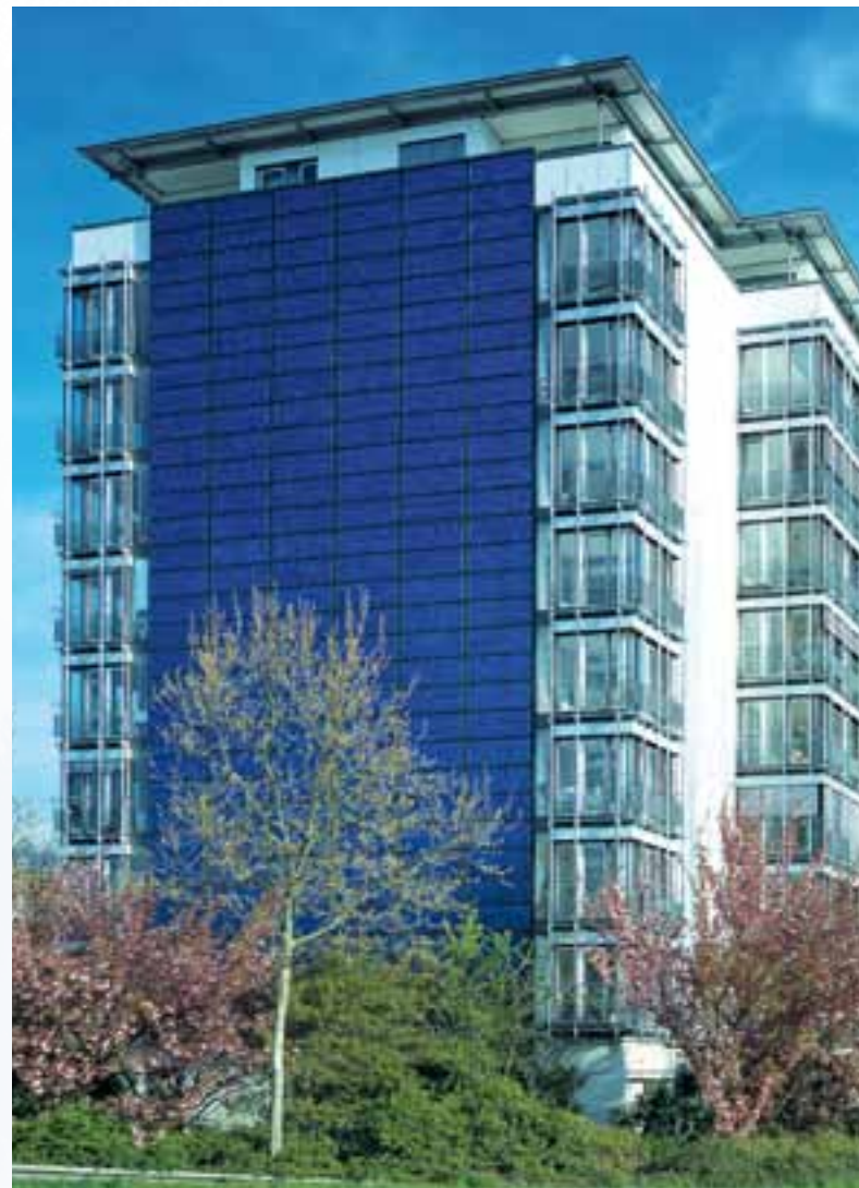
Solar facade of the residential complex at Wilmersdorfer Street
