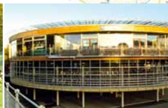
Bicycle station 'Mobile' at the main station
