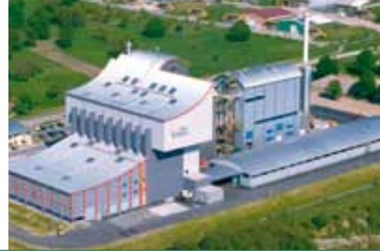
Thermal waste treatment plant generating energy from non-recyclable waste, Industrial Park Breisgau
