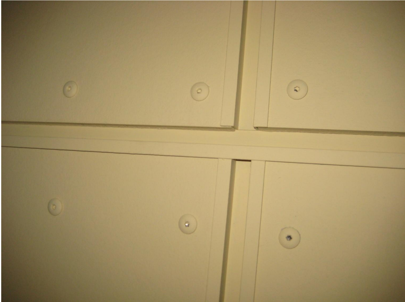
Detail of joints at cement board mock-up panel.
