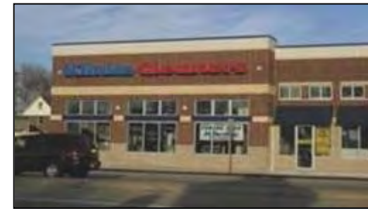
FIGURE 4.10 Windows at street level, awnings, and quality materials are all design elements that should be considered during redevelopment
