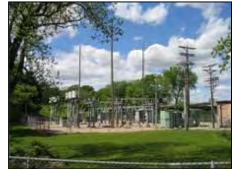
FIGURE 2.34 MG&E Power Station on Spring Harbor Drive
