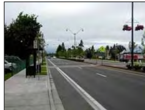
FIGURE 4.18 Separate facilities for transit users, pedestrians, and bicyclists make this an active arterial for many users.
