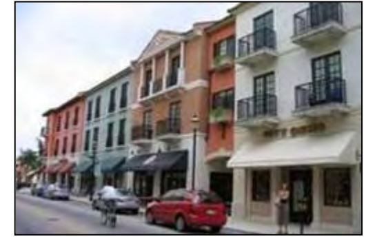
FIGURE 4.6 Façade variation and attention to detail, such as balconies and awnings, help to break up the mass of a large building
