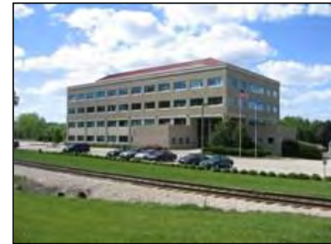
FIGURE 2.19 The Erdman Holdings Campus on Old Middleton Road and Whitney Way
