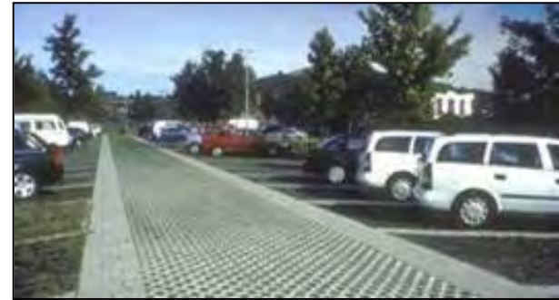
FIGURE 4.14 Permeable surface parking lot that incorporates stormwater
