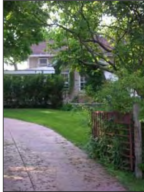
FIGURE 2.28 Hickory Hill House (1842) built by John G. Hicks. Presently (2006) owned by Daniel W. Erdman.
