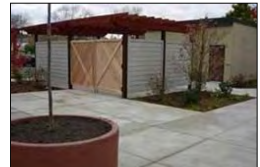
FIGURE 4.8 Simple structure to hide trash bins can make a large aesthetic difference
