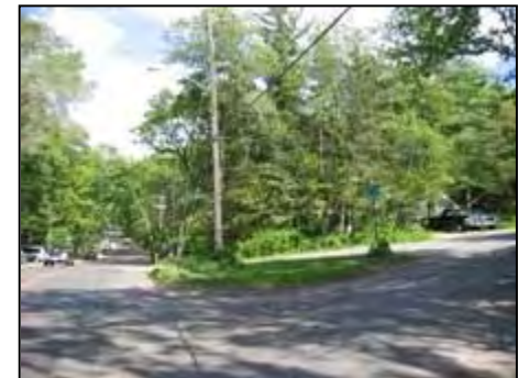
FIGURE 2.35 Utility Lines along Lake Mendota Drive
