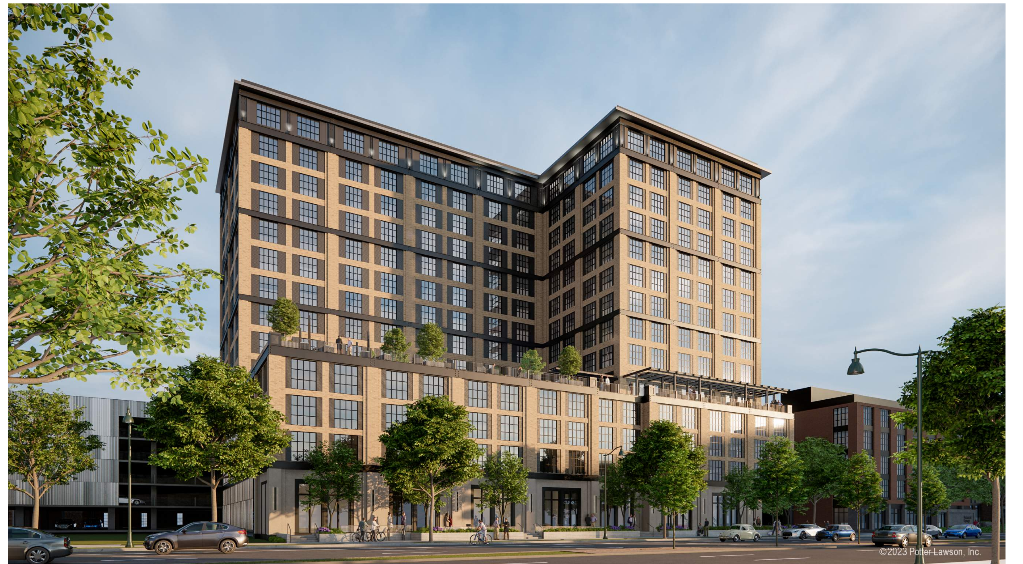
GROUND-LEVEL VIEW FROM BREARLY AND EAST WASHINGTON
