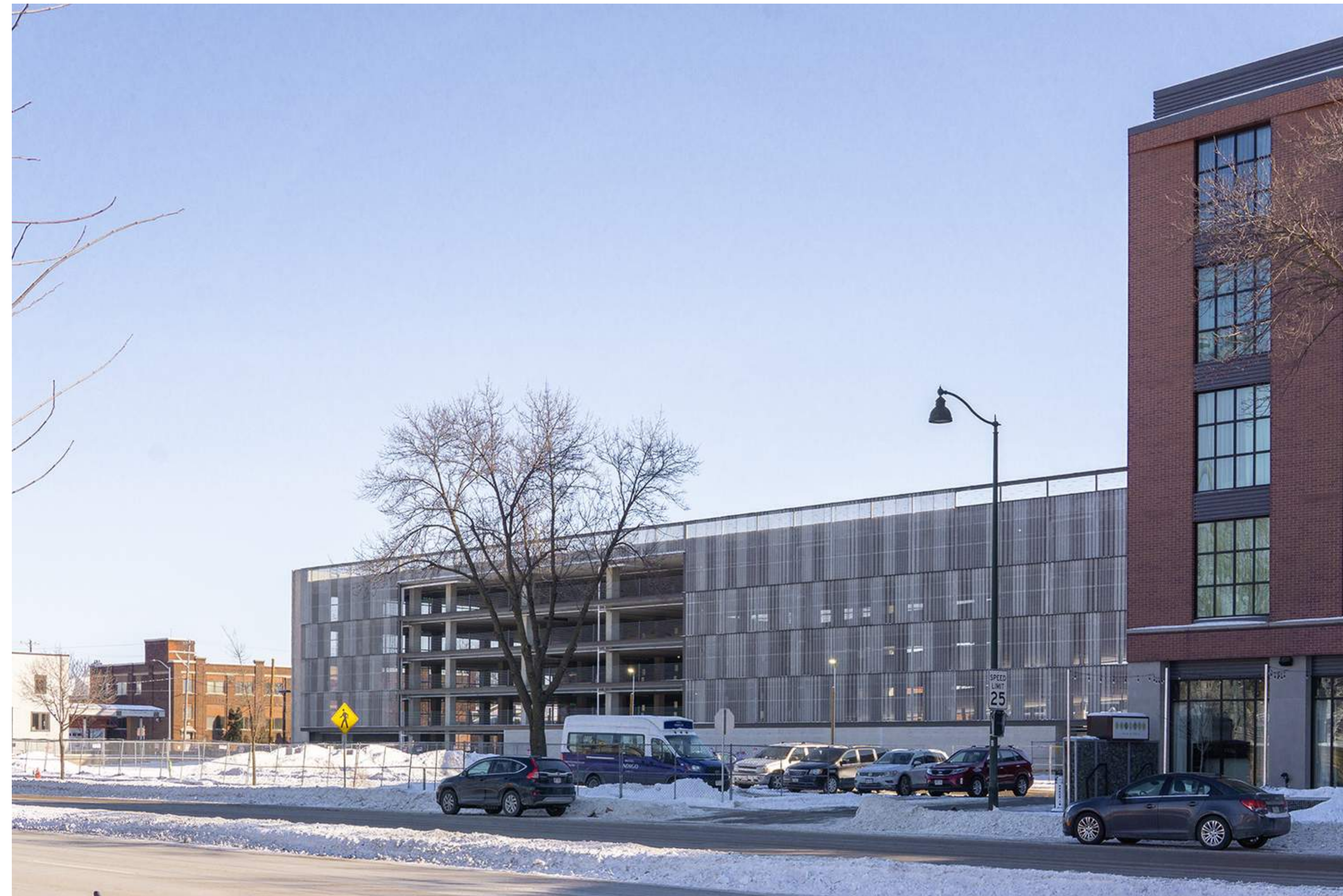
Project site along E. Washington Ave. (Phase 1 Parking Ramp is visible in background)
