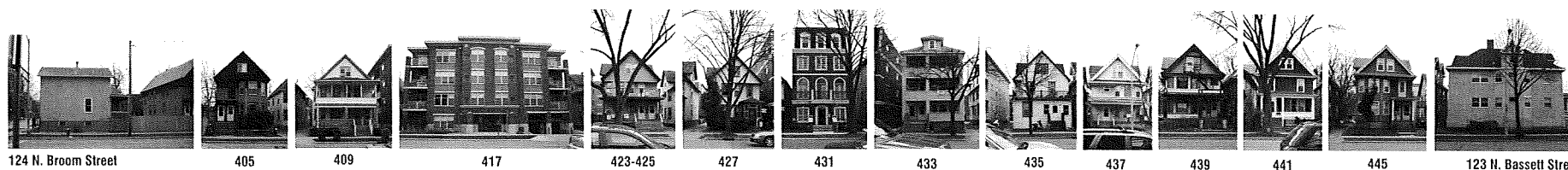
3 EXISTING STREETScape AT OPPOSITE SIDE OF W. DAYTON ST D101
