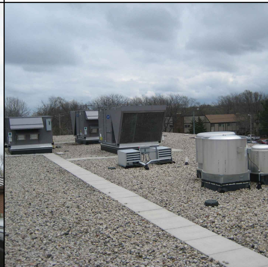
EXISTING BUILDING ROOFTOP
