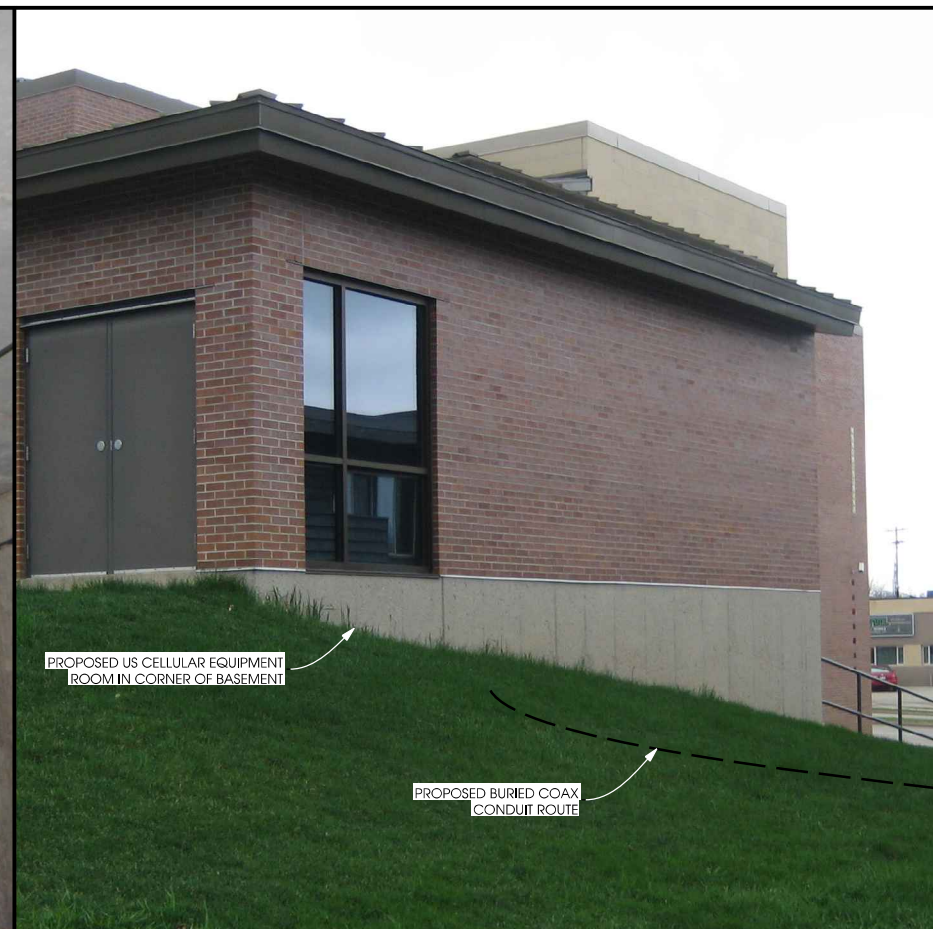
OUTSIDE EQUIPMENT ROOM
