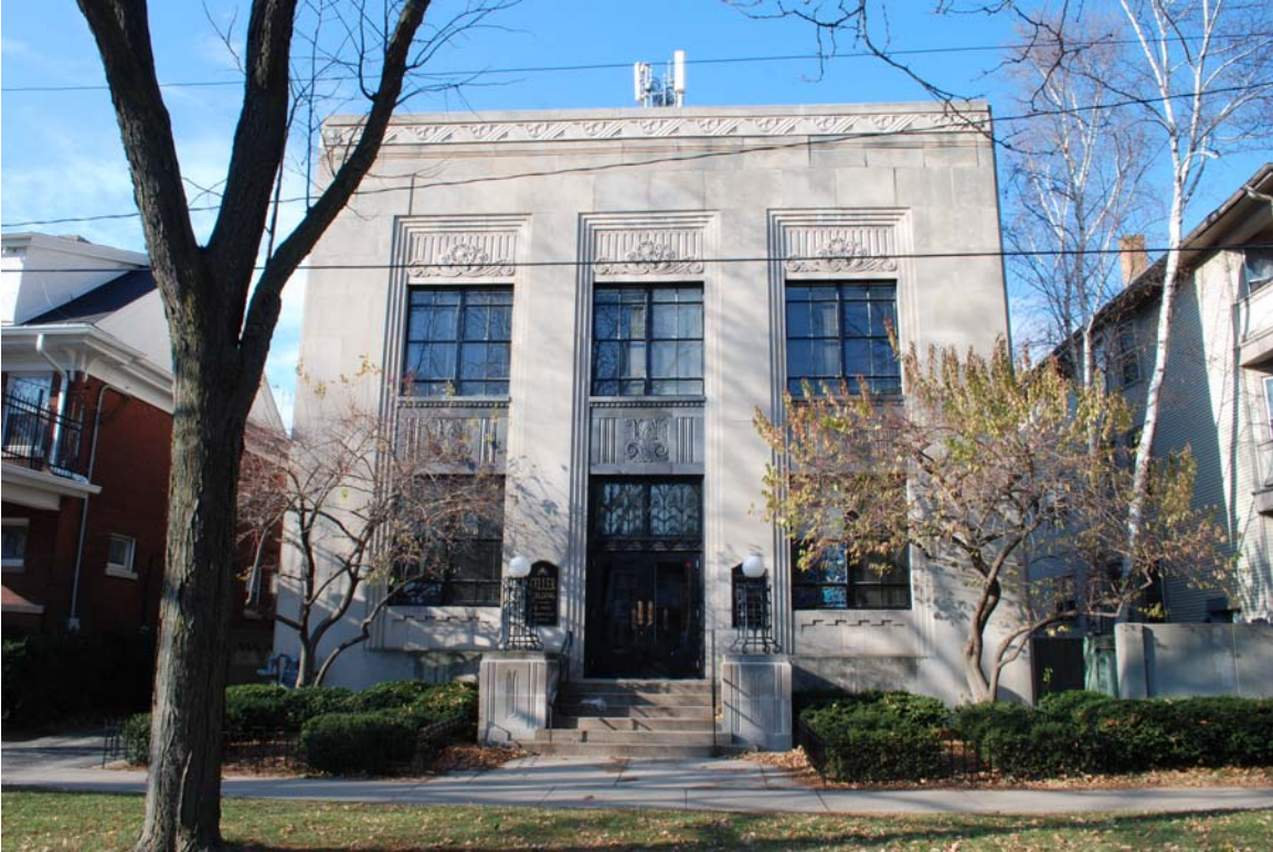
Holstein Friesian Association Building, 448 West Washington Avenue
