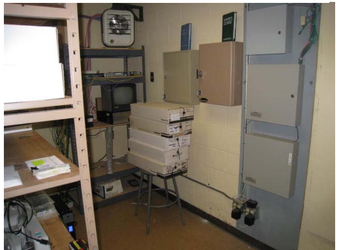
Photo 15: Utility Room / Storage Closet (Basement Level)
