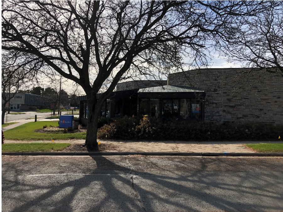
Photo 1: Northerly Façade (View from Vernon Boulevard)
