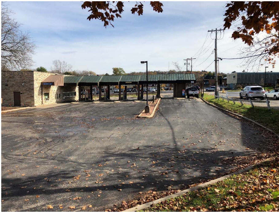
Photo 4: Drive-Thru Canopy (View from Drive-Thru Lane Area)
