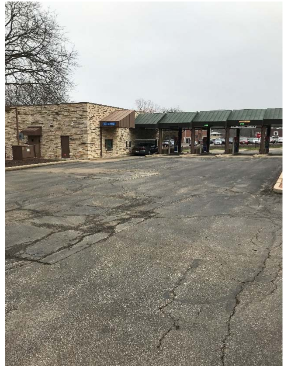
Photo 3: Westerly/Southerly Façade (View from Drive-Thru Lane Area)
