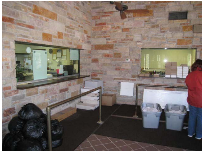
Photo 7: Teller Windows Counters (Main Lobby Area)
