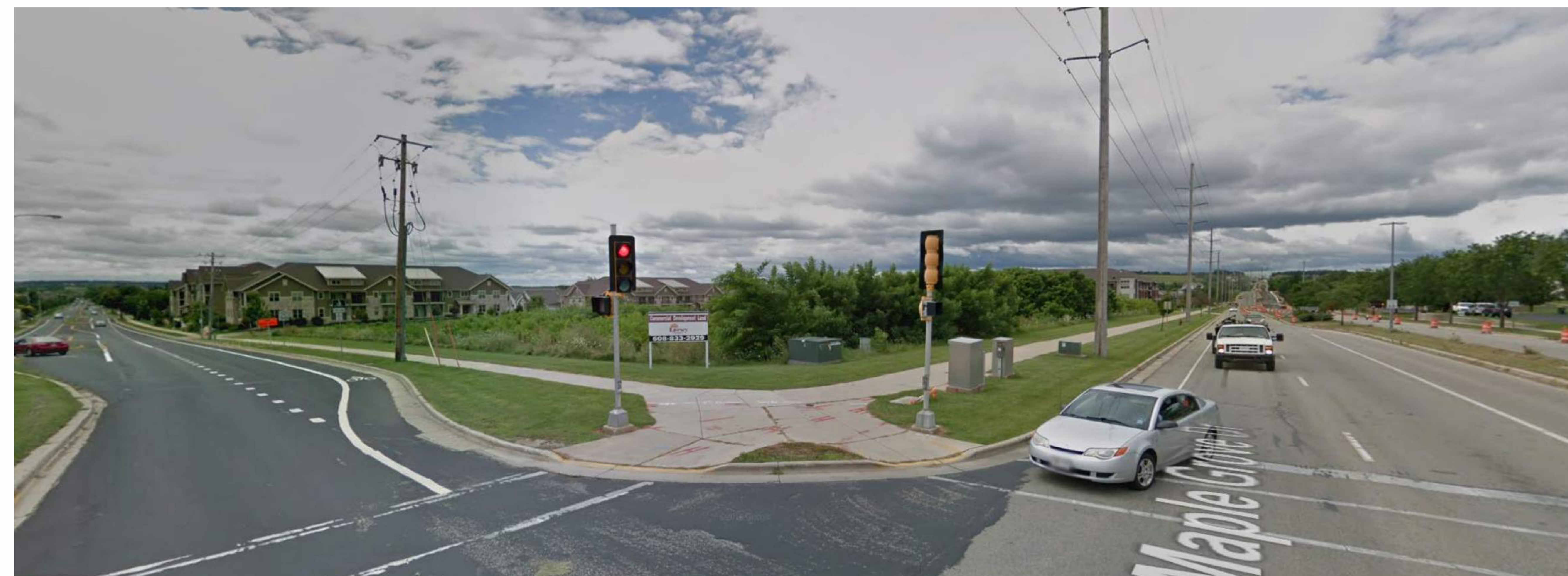
NORTHEAST CORNER - McKEE RD & MAPLE GROVE DR (SITE CORNER)
