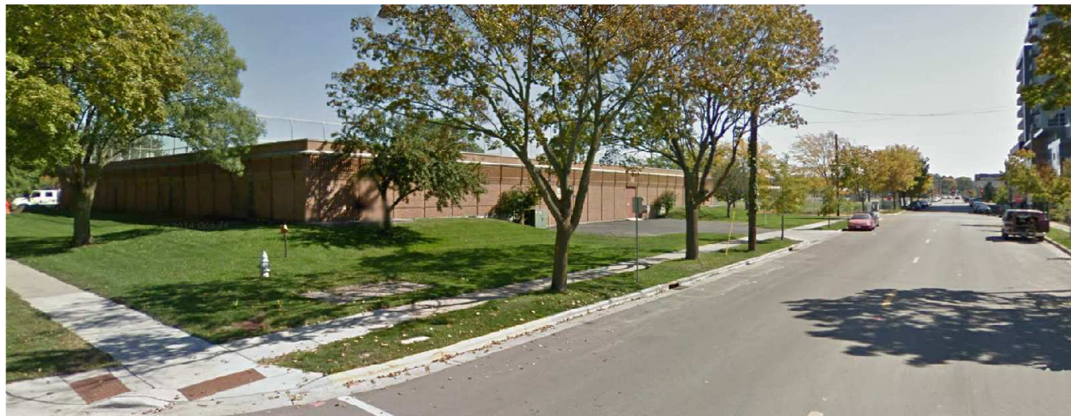
REYNOLDS PARK TENNIS COURTS AND WATER TREATMENT BUILDING ACROSS LIVINGSTON
