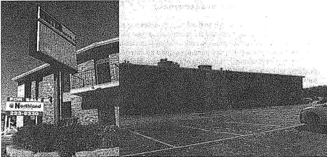
Exterior photographs of existing South and West building elevations
