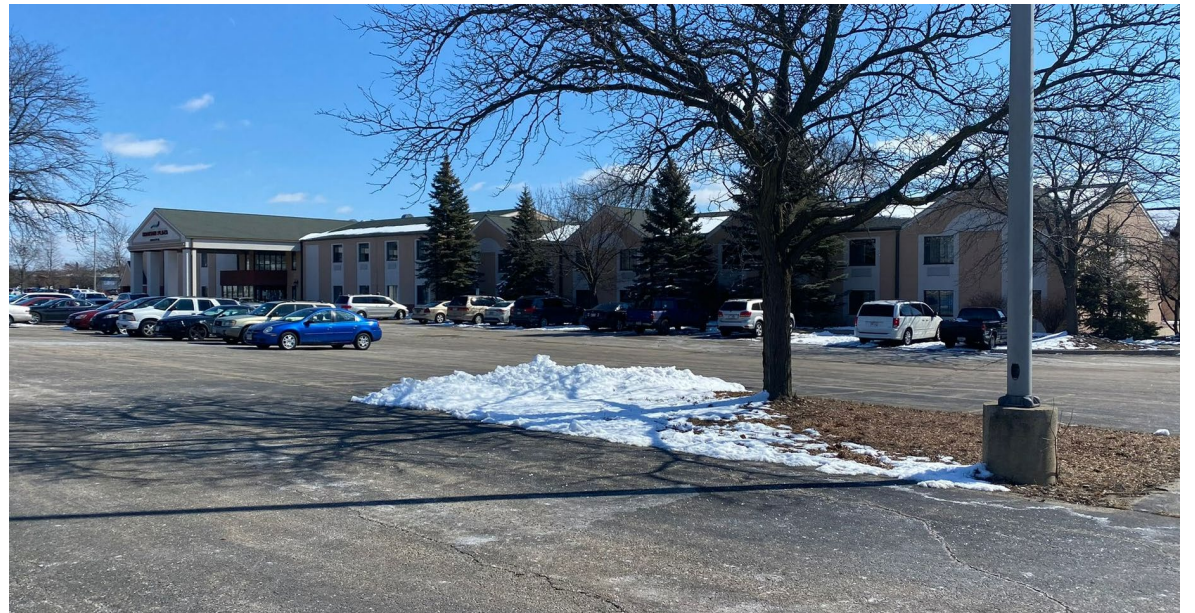
Plato's Madison - Photos of Existing Site
