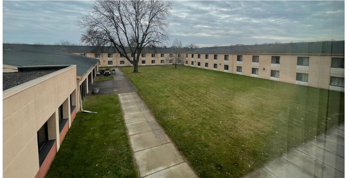
Plato's Madison - Photos of Existing Site
