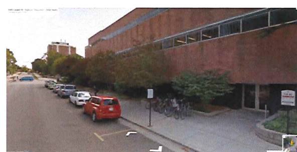
Basement entry under first floor cantilever, looking east
