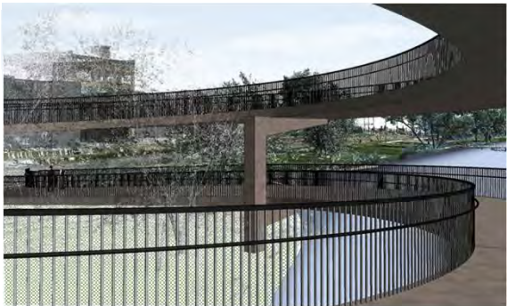
The pier supporting the pedestrian bicycle overpass ramp can be cantilevered, yet some of the structure would still extend over the lake..
