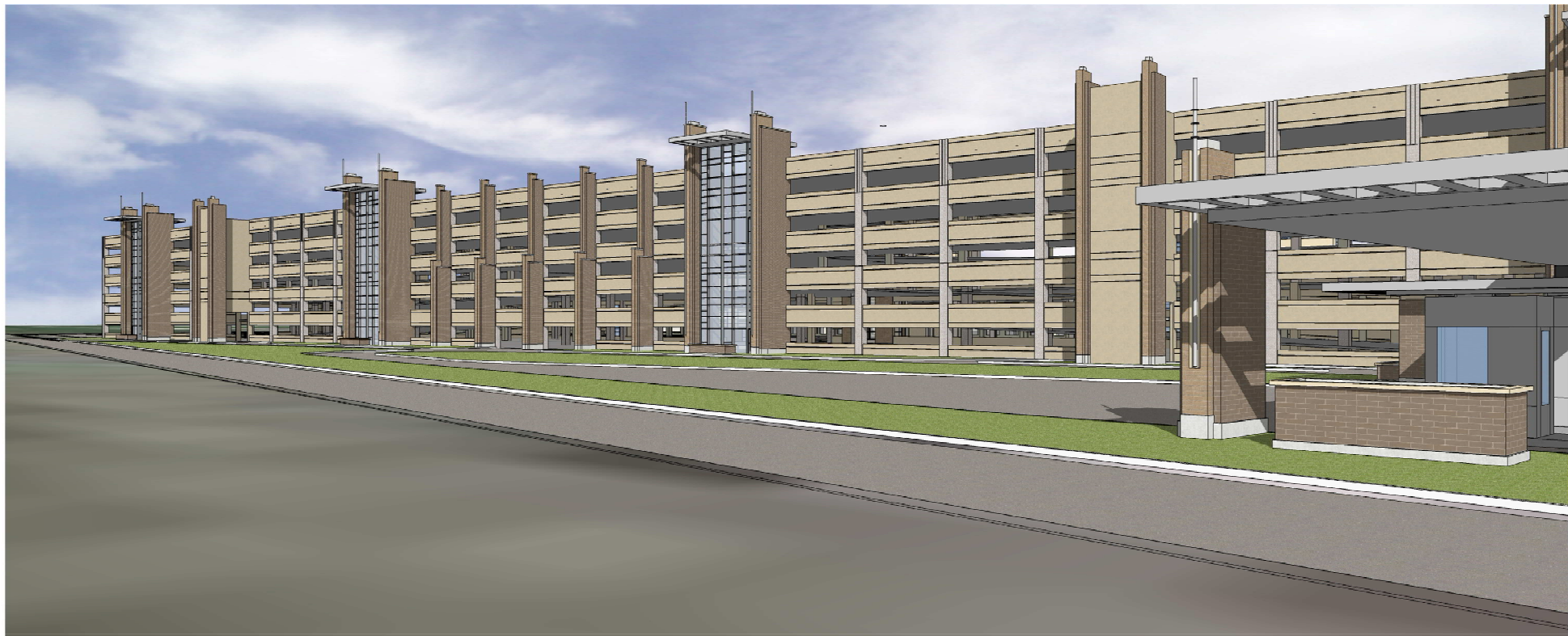
View From West
