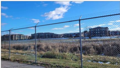
8' GALVANIZED CHAINLINK W/ BARBWIRE (C)
