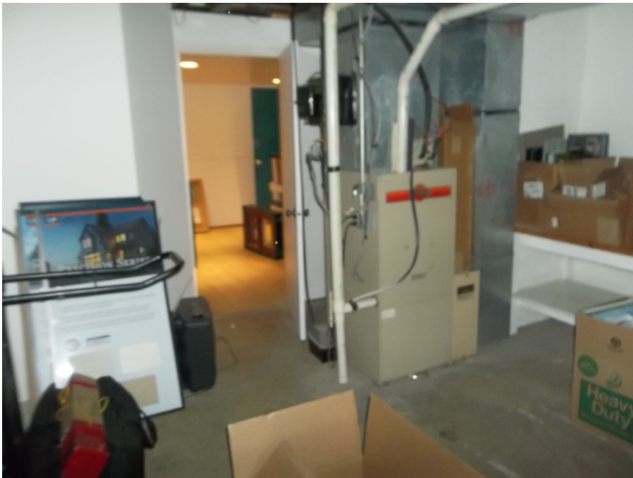
Basement Area Interior of Building
