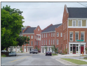
Fig. G4-7: Housing at Town Square.
