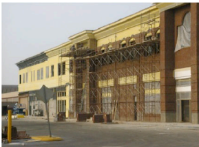
Fig. G2-10: Turning the Mall Inside Out: two story office from blank wall of former department store.
