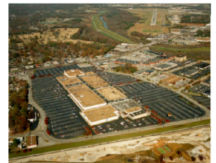
Fig. G2-1: Aerial View, Eastgate Mall prior to renovation.
