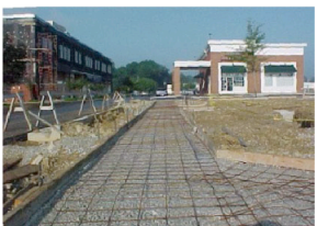
Fig. G2-12: Brainerd Town Square, under construction in 1999.
