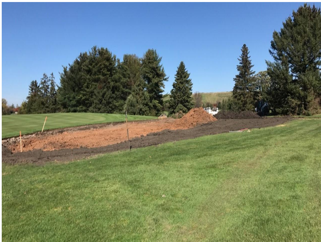
Yahara bunker project East Course Hole # 11
