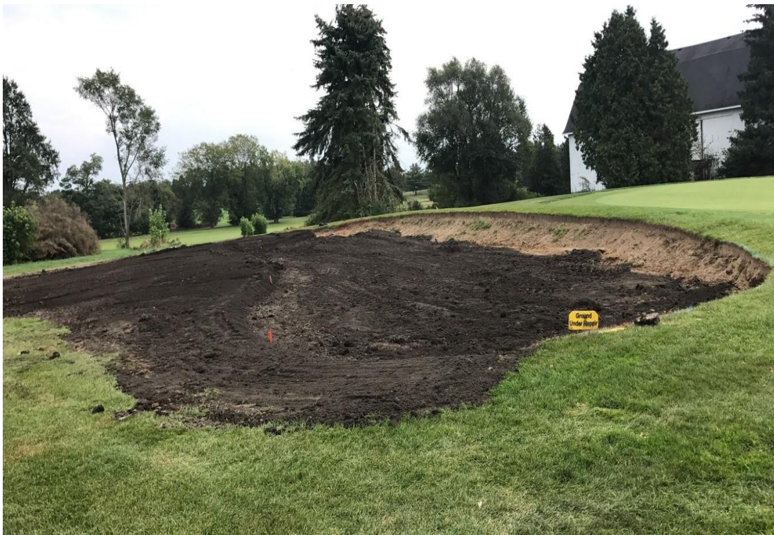
Yahara bunker project West Course Hole #2
