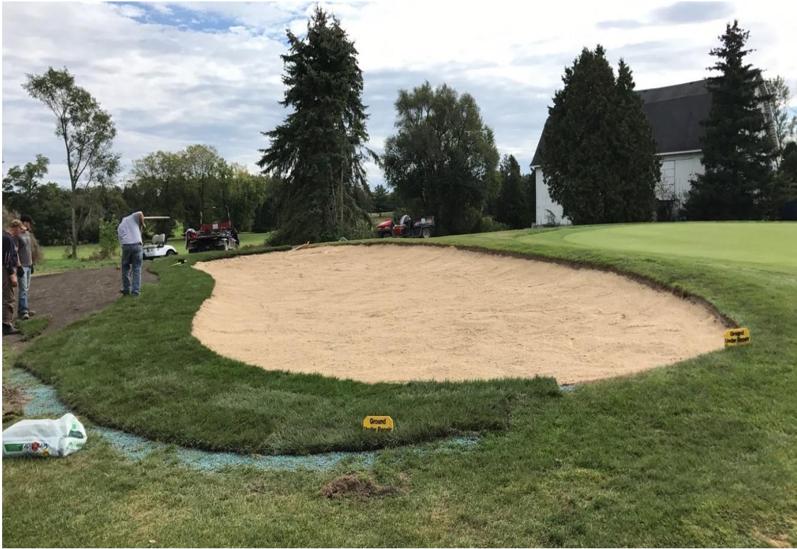
Yahara bunker project West Course Hole #2
