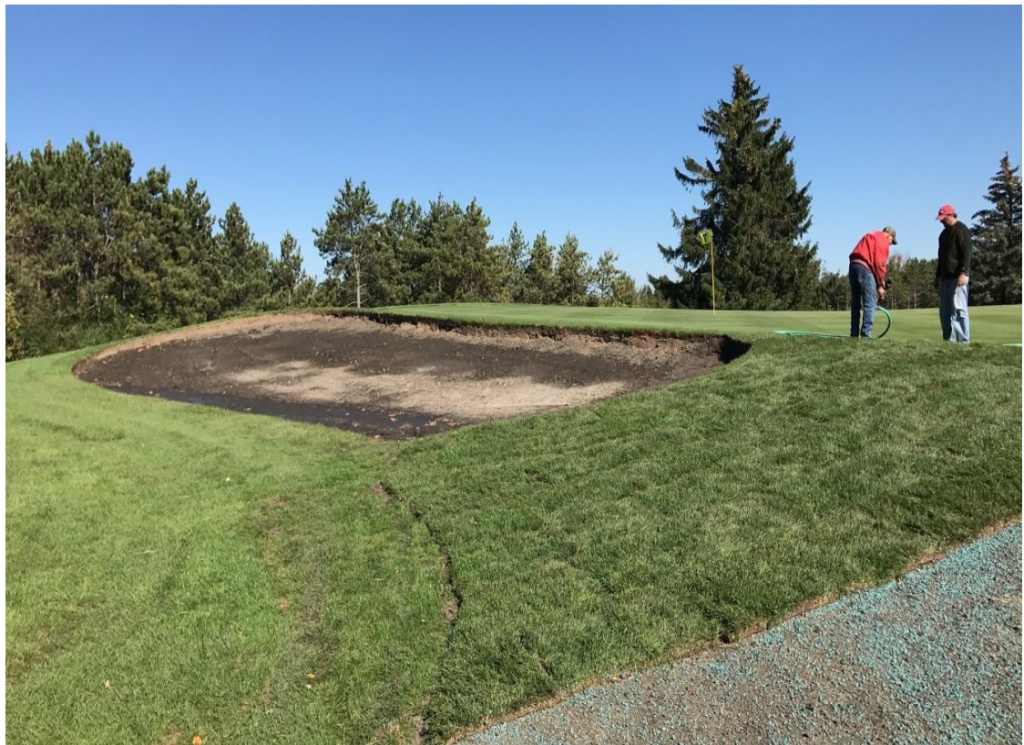
Yahara bunker project West Course Hole #7
