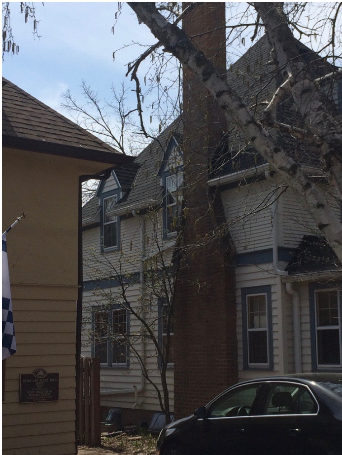
Northeast exterior (replace 2 uppers only)
