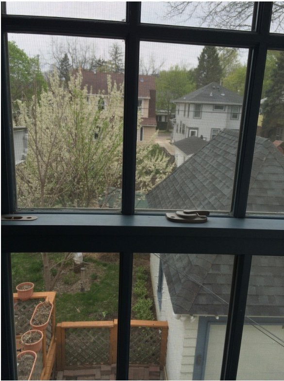
Newer Anderson window in remodeled bathroom
