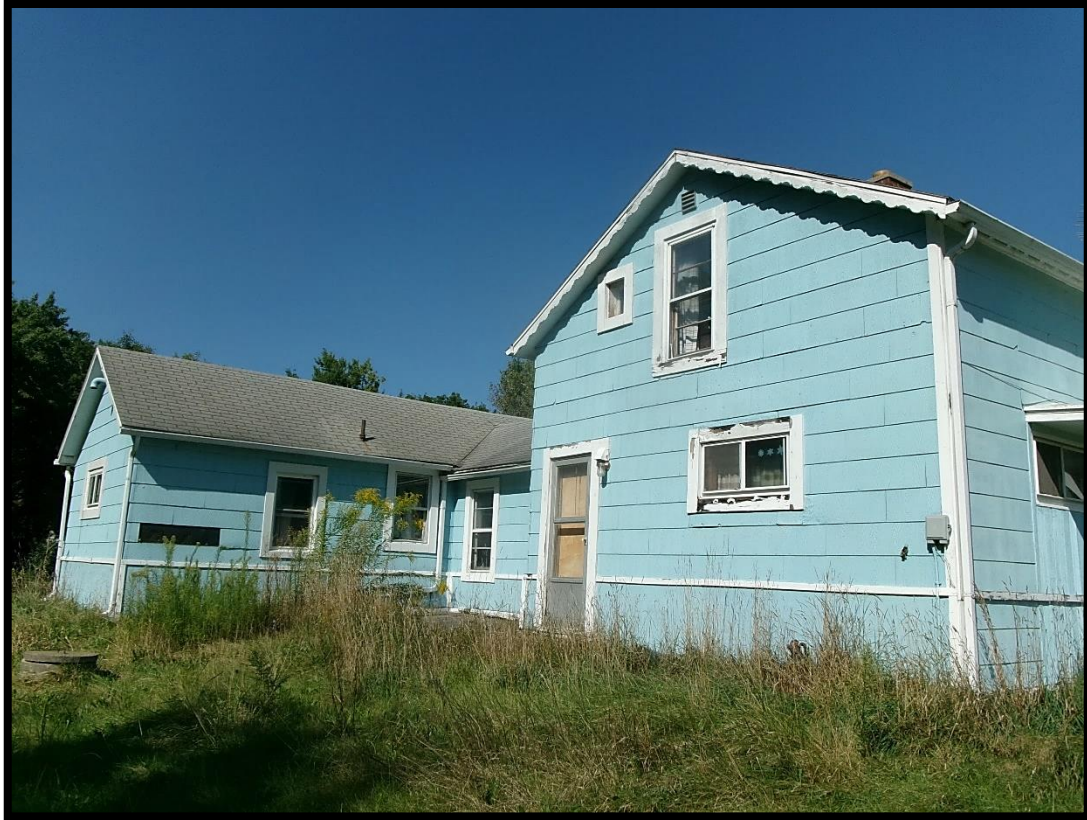
HOUSE - TO BE DEMOLISHED
