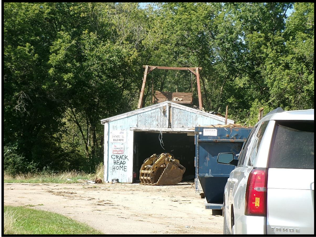
GARAGE - TO BE DEMOLISHED
