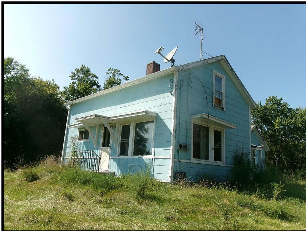
HOUSE - TO BE DEMOLISHED
