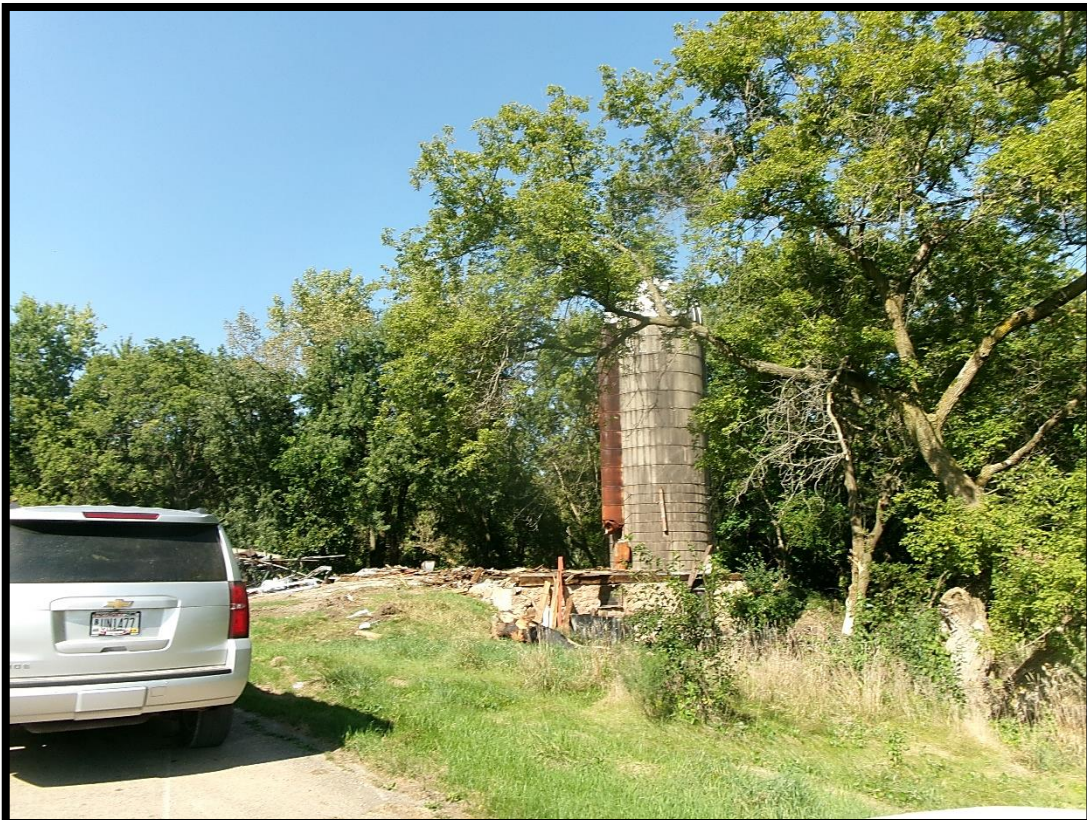
BARN FOUNDATION & SILO
