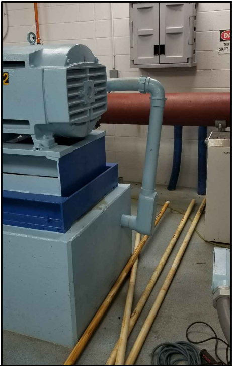
ELECTRIC SUPPLY CONDUIT
