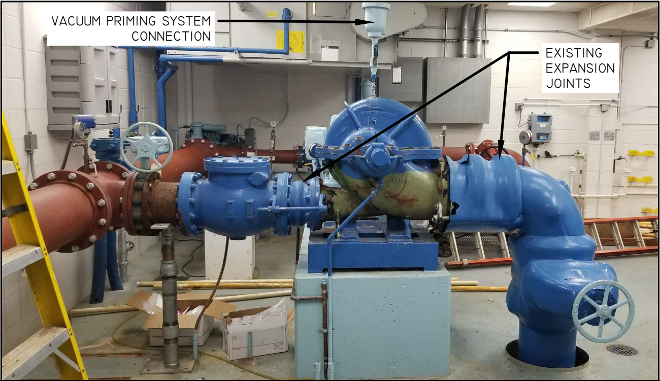
BOOSTER PUMP #2 SIDE VIEW / PUMP SIDE
