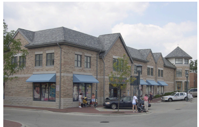
Fig. D-3: Pedestrian routes should be clear and direct users to additional destinations within the site
