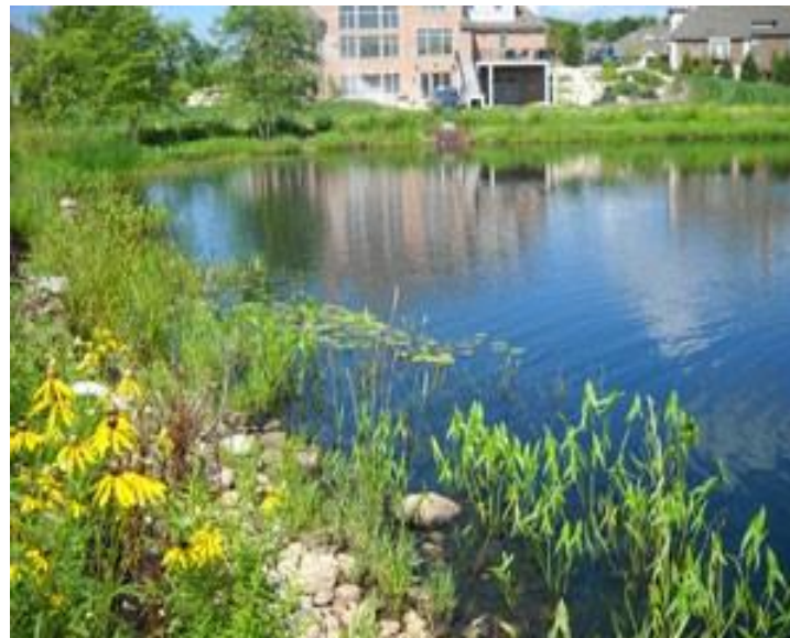
Stormwater Detention Ponds
