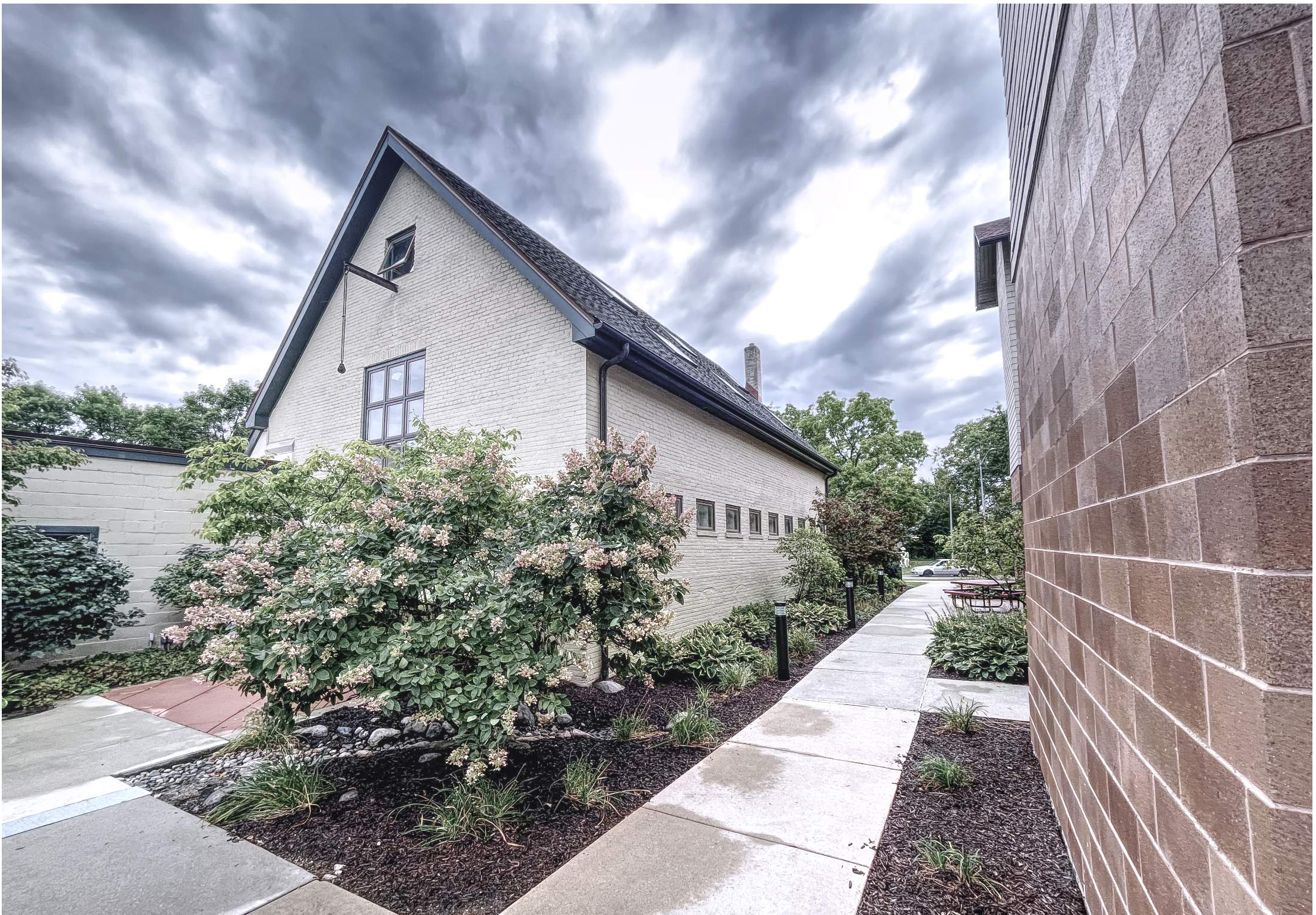
Existing | Front Entry
