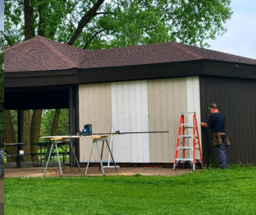
Marlborough Park shelter
