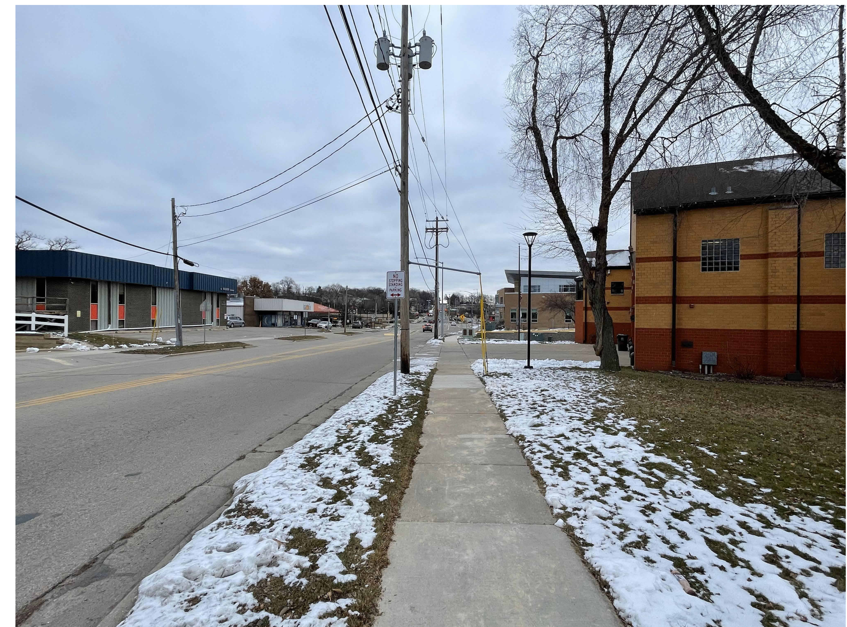
View from Intersection of Pertt Street and West Badger Road Looking East at Madison Fire Station #6
