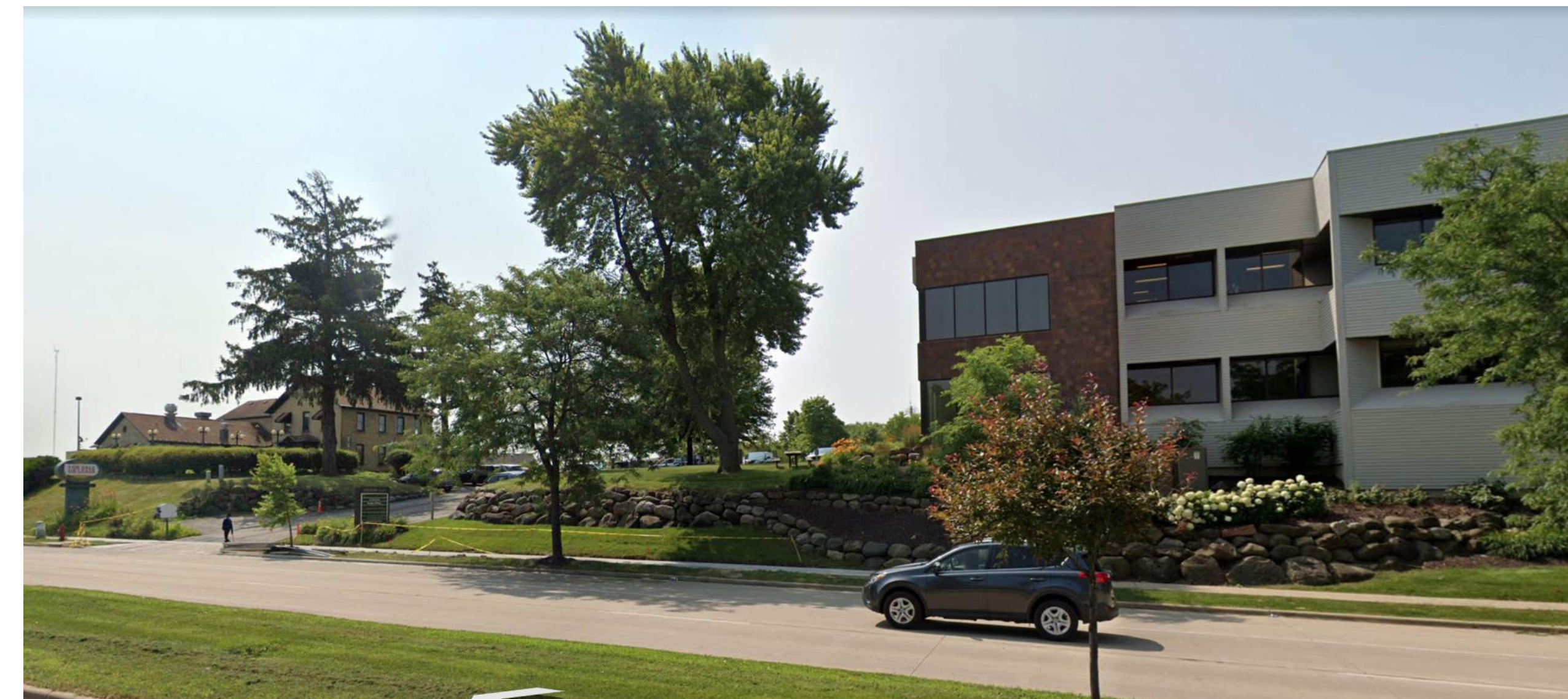
Building west of site along Mineral Point Rd.
