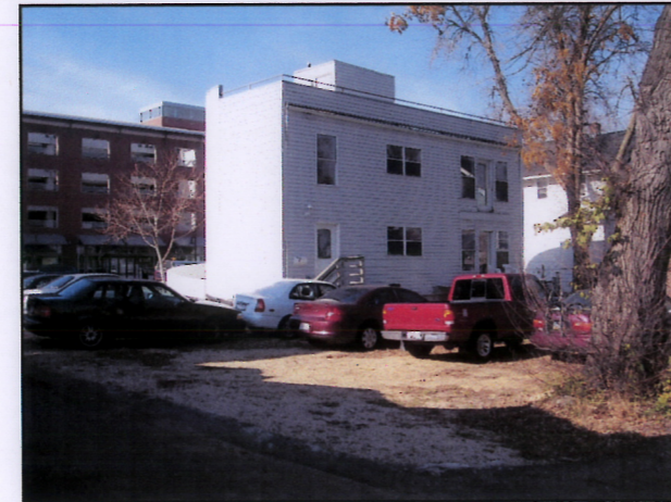
CENTER OF ALLEY LOOKING NORTHWEST
