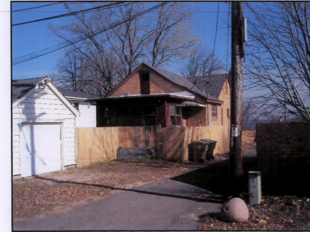
CENTER OF ALLEY LOOKING NORTHEAST
