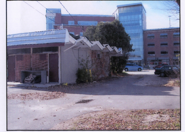
NORTHEAST CORNER OF LOT LOOKING SOUTHWEST
