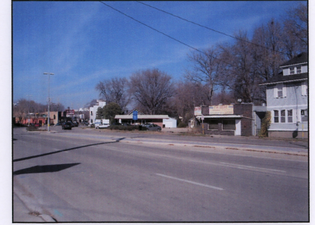
SITE VIEW FROM SOUTHWEST
