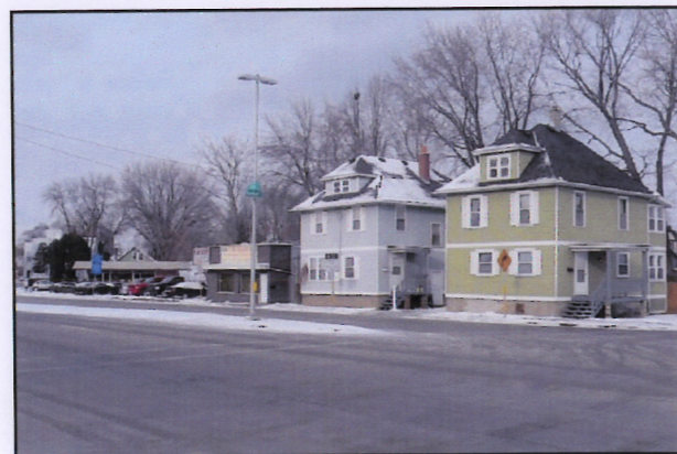
SITE VIEW FROM SOUTHWEST
