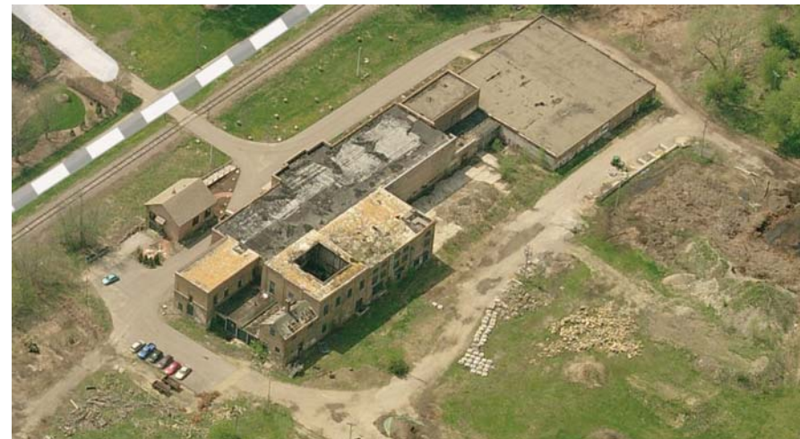
EXISTING NORTH FACADE AERIAL
