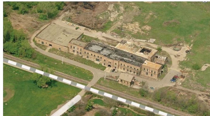
EXISTING SOUTH FACADE AERIAL
