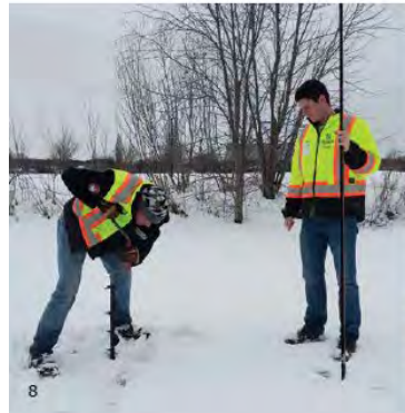
Fitchburg employees core through the ice at one of the city's water quality ponds to measure the depth of water and soft sediment. When there is less than 3.5 feet of water, dredging is done to remove buildup, which helps ensure the ponds can effectively clean water by allowing suspended solids (including attached phosphorus) to settle out.
