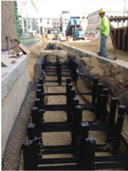
Figure 2 Deeproot's Silva Cells Installation
