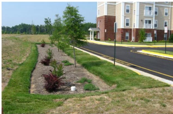
Vegetated filter strip at the edge of a parking lot intercepts and filters stormwater runoff before the water reaches the infiltration bed at the center of the practice.
