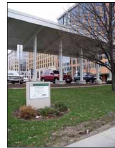
A solar canopy
