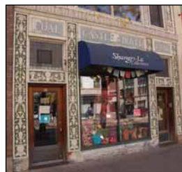
Castle & Doyle Building
