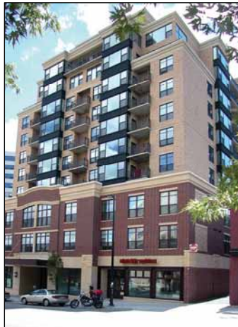
The Madison Mark incorporates stepbacks above the third story
