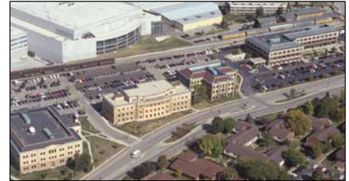
A bird's eye view of the West Rail Corridor, with Regent Street in the foreground
