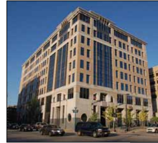
Risser Justice Building
