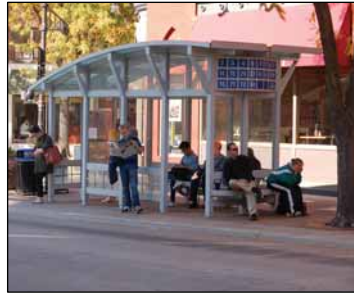
State Street bus shelter
