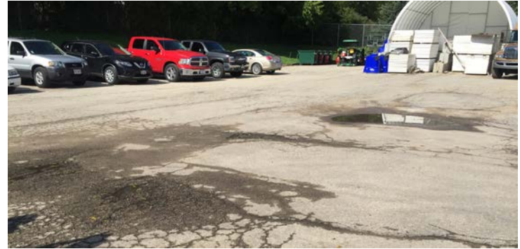
Summit Maintenance Facility Parking Lot
