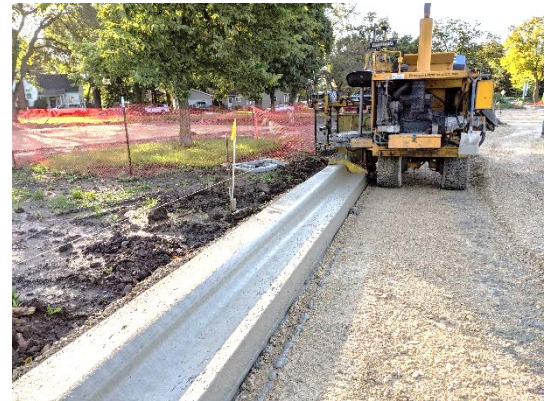
Olbrich Park Walter Street Parking Lot
