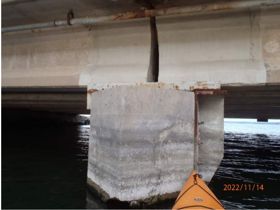
Photo 3: Typical bearing bracket assembly
