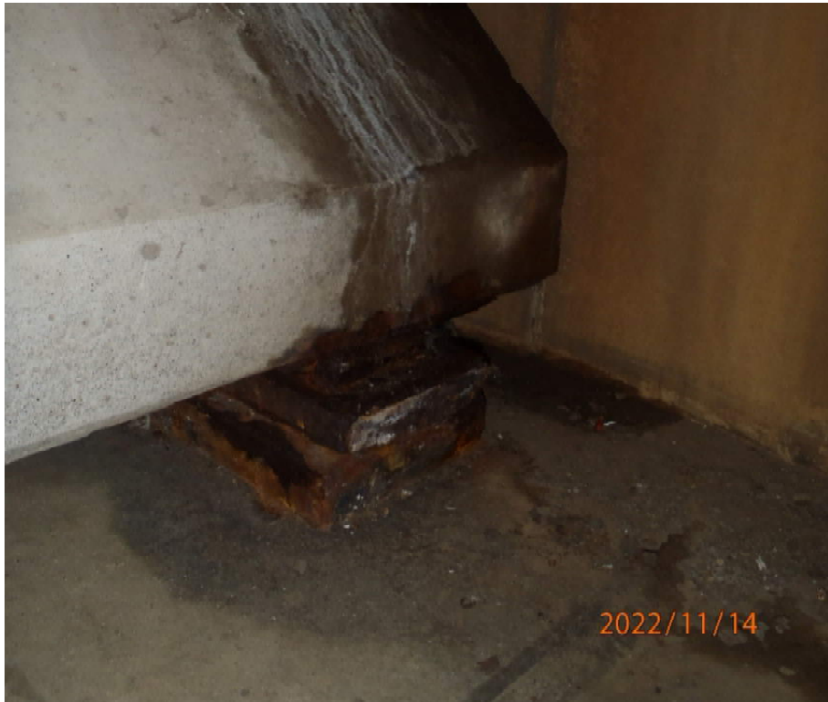
Photo 4: Typical expansion bearing
