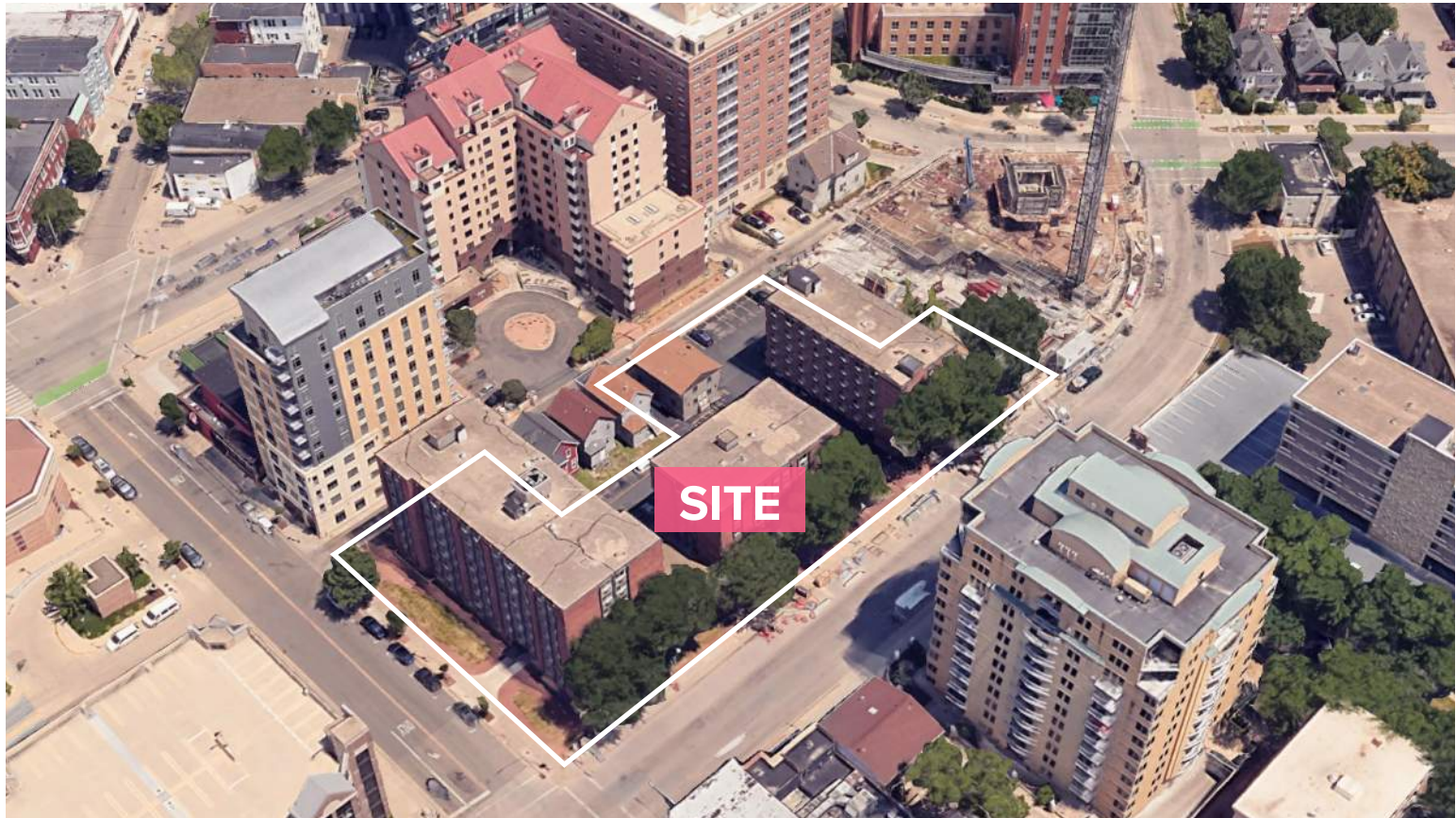
AERIAL FROM SW
