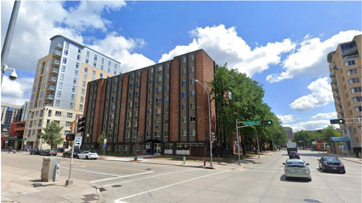
FRANCES & JOHNSON INTERSECTION
