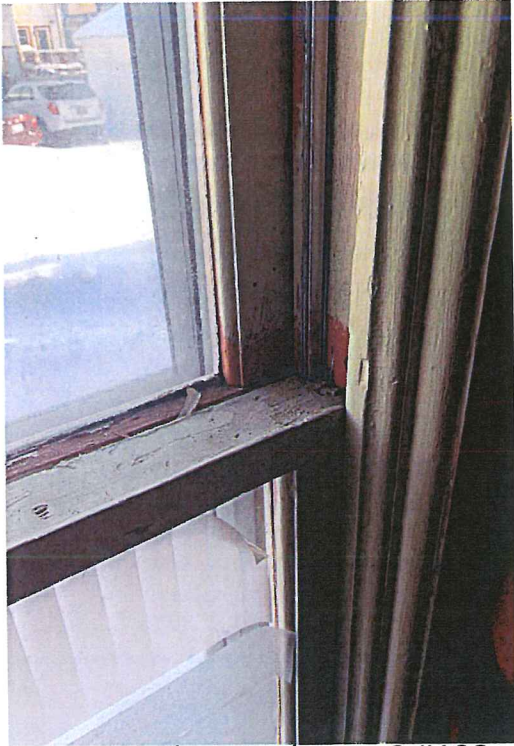
1st Floor Bedroom 2 #108
