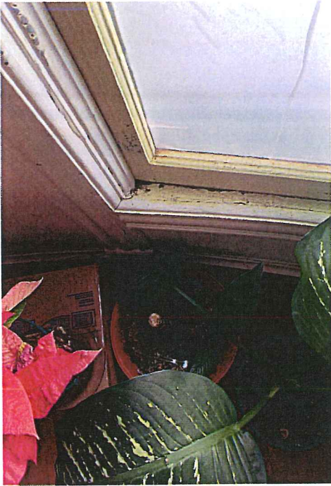
1st Floor Bedroom2 #107
