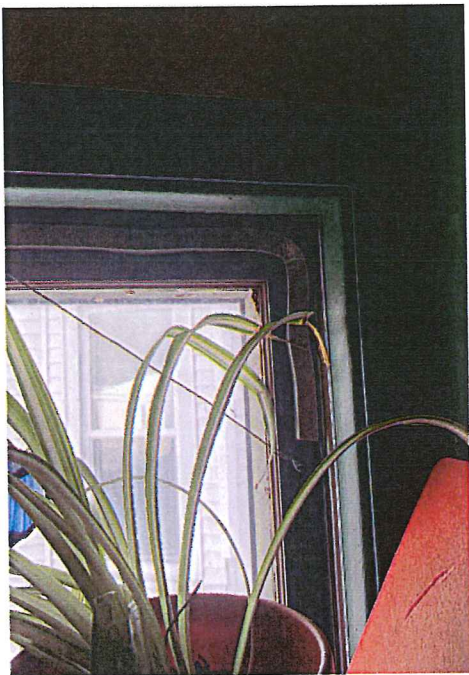
1st Floor Bedroom 2 #109
