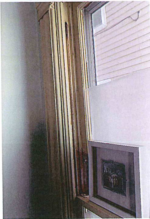
1st Floor Bedroom 2 #107
