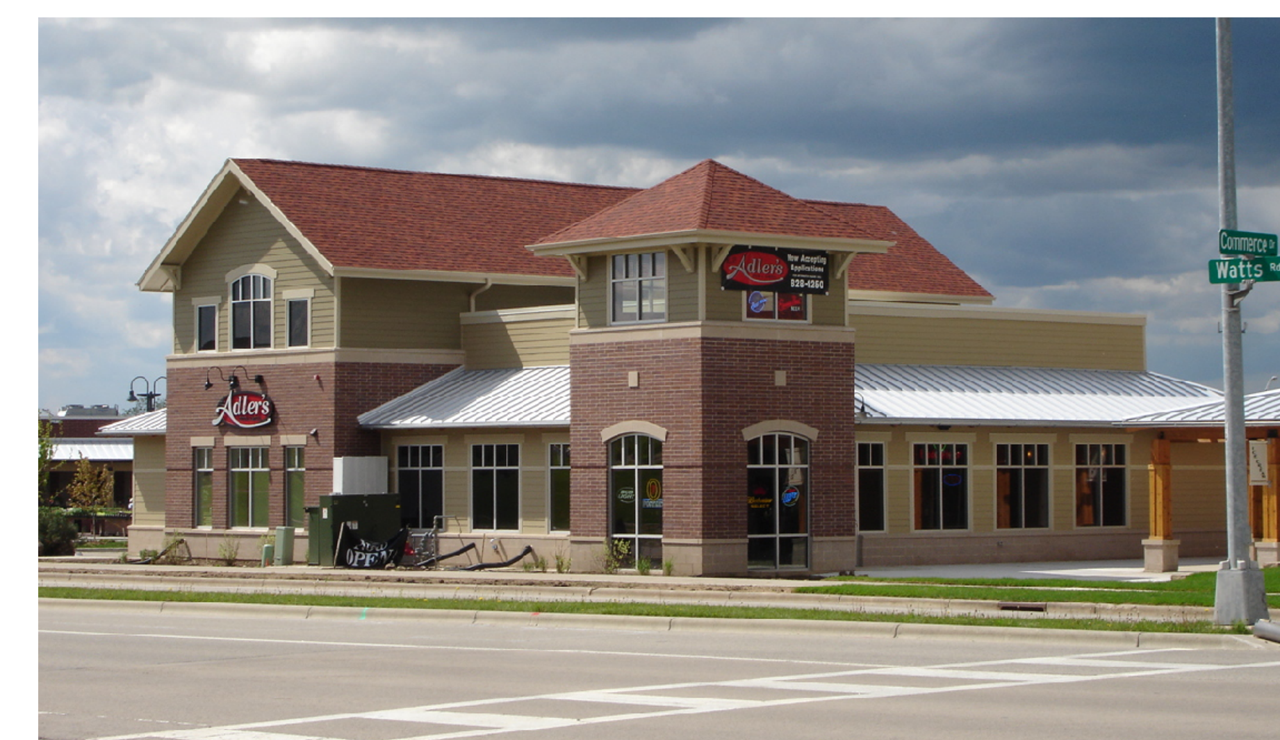
RETAIL SPACE ON WATTS ROAD
