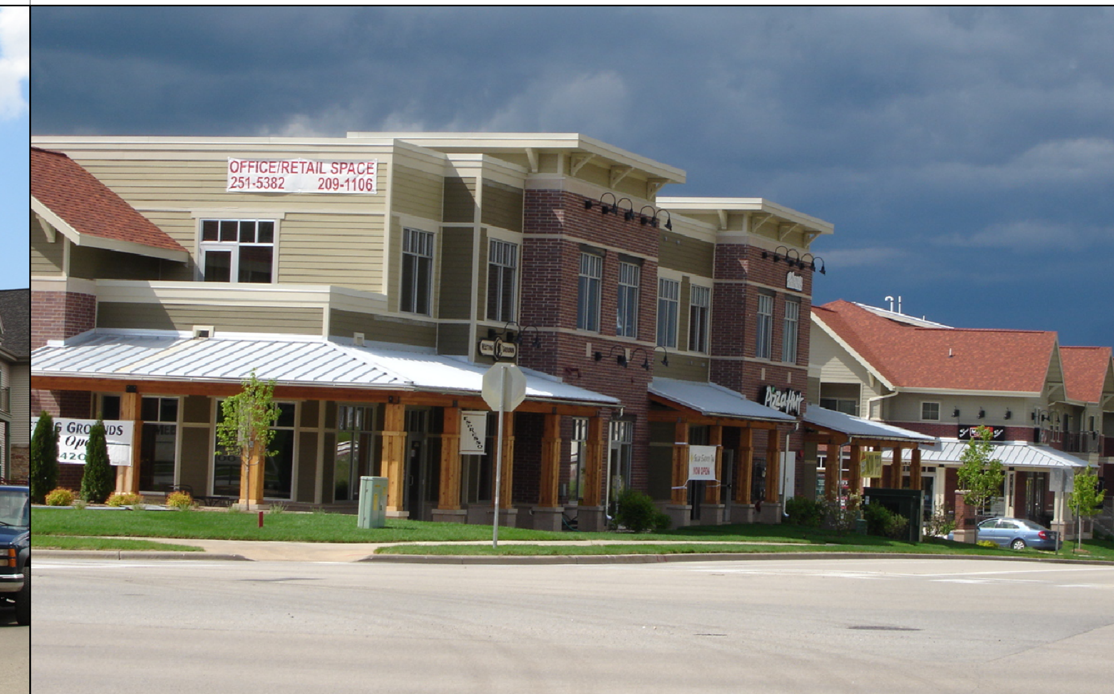
RETAIL SPACE ON WATTS ROAD
