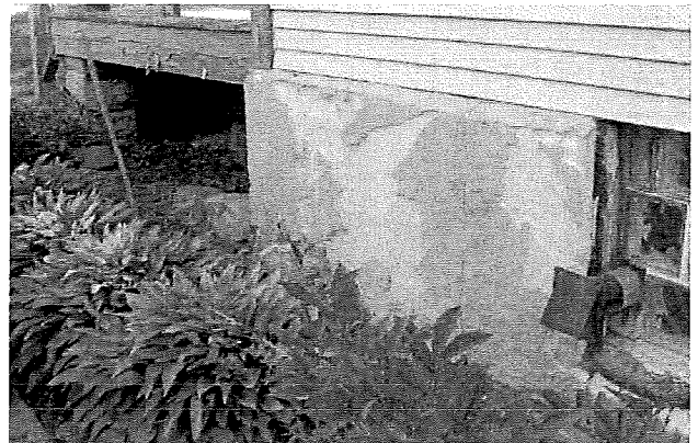
315 S. Mills St. CONDITION EXAMPLES EXTERNAL FOUNDATION WALL- SOUTH SIDE
