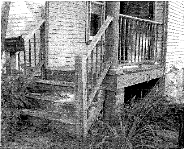
315 S. Mills St. CONDITION EXAMPLES FRONT PORCH
