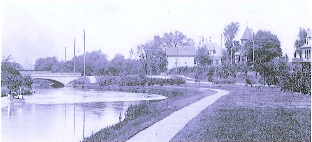
Dr. Hurd House and clinic, c. 1910, looking along Yahara River Parkway across Winnebago Street. Photo: Wisconsin Historical Society, by Charles N. Brown, Image ID 3956.
