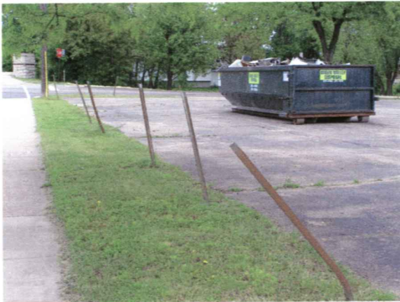
1451 East Washington Avenue Dangerous Posts Near Sidewalk Unscreened Trash Container May 28, 2005
