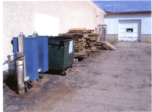
1433 East Main Street Trash Equipment Stored Outside Visible to Street Deteriorated Door Rusted Roof May 28, 2005
