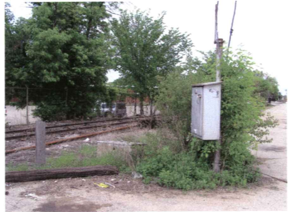
1422 East Washington Avenue Abandoned Railroad Structure Old Ties May 28, 2005
