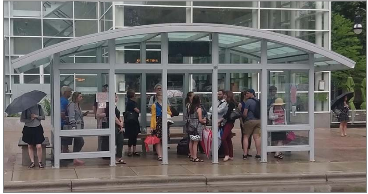
Figure 4-3 Bus Shelter Capitol Square
