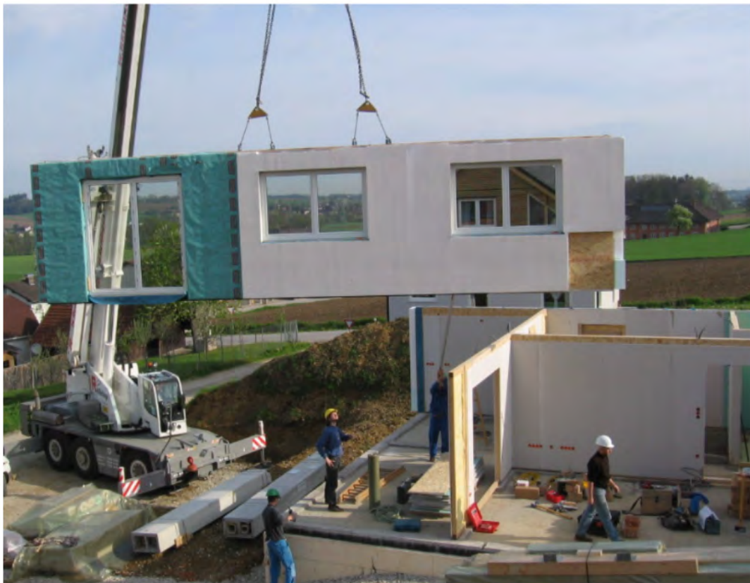
Modular housing being transported to the build site
